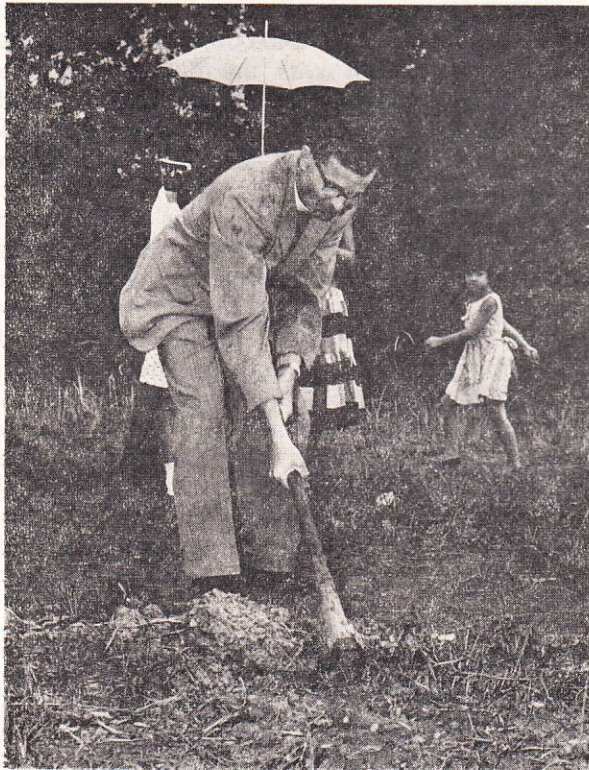
The breaking of the ground by Rev. Christopher Smith for the building of the proposed Trinity Methodist Church.
